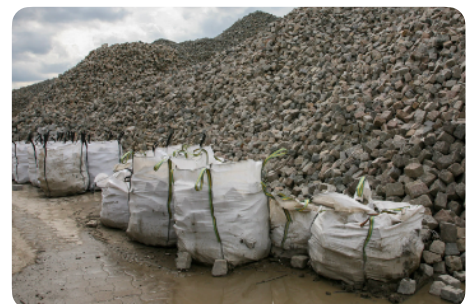
Storage of paving stones in big bags
