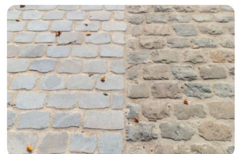
Installation of sawn / rough pavers
