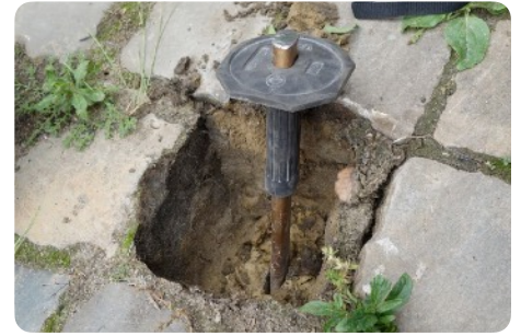
Sandstone setts and traditional laying on a sand bed: recovery is generally easy
