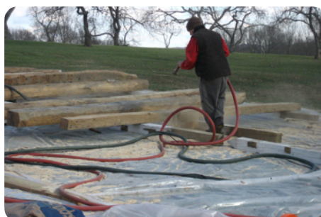
Reiniging van hout © yr-architecture
