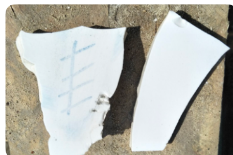
"Porous" glaze vs glaze in good condition
