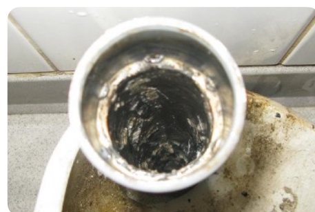
Partially cleaned drainage device
